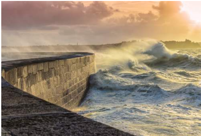
Photo 3. Sea Wall. Low maintenance cost. High cost per metre, £700 – £5,400.
